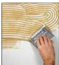
Apply Marlite Brand Adhesive to the back of panels and apply them to a subwall.
